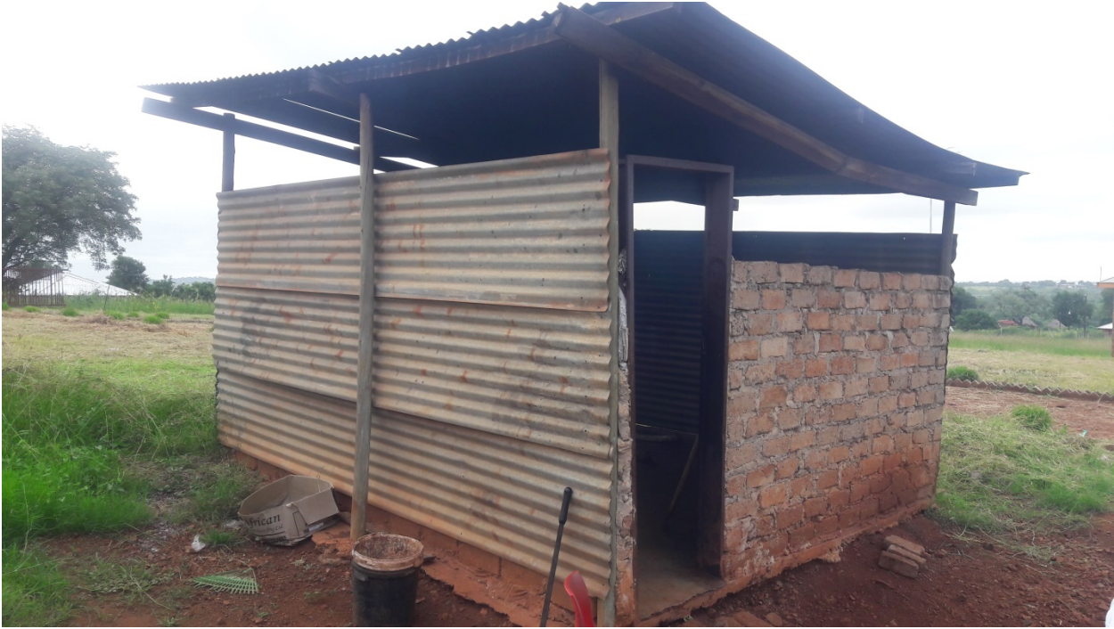
The dilapidated shack which was in use
